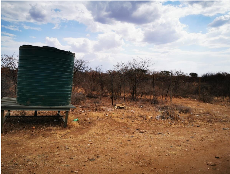
Figure 35: Jojo tank used by small community on the R525 between Mopane and Bokmakirie
