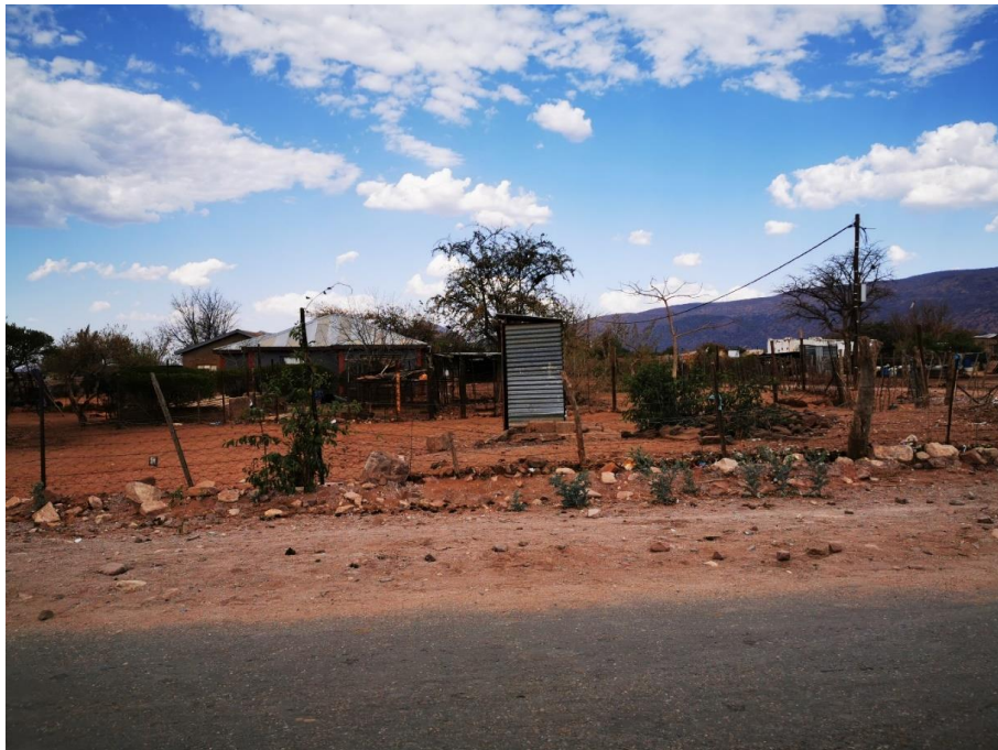
Figure 34: Pit latrine in Mudimeli
